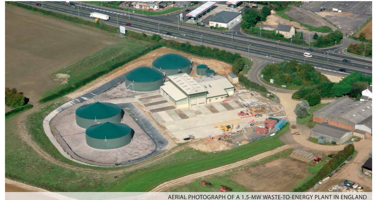
AERIAL PHOTOGRAPH OF A 1.5-MW WASTE-TO-ENERGY PLANT IN ENGLAND
